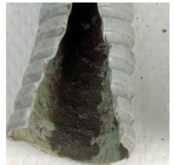
Biofilm in the hose of the suction unit
